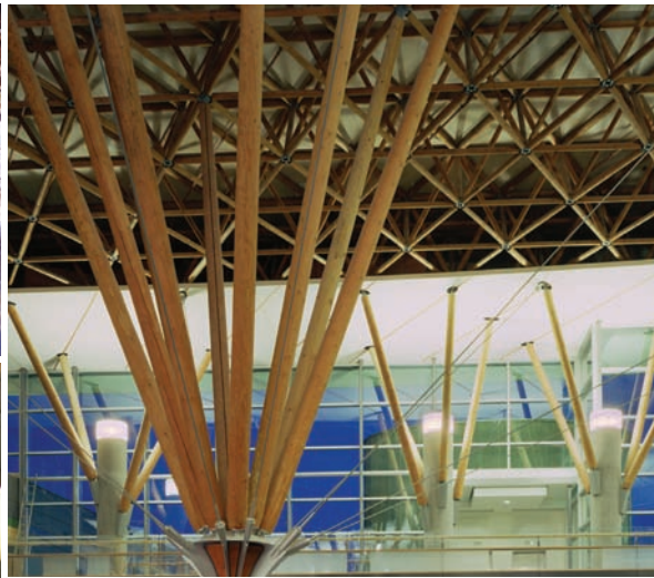
Bing Thom Architects, Surrey_short list captions_wood . (15, 18) Peeler core processing and assembly techniques for Surrey City Center atrium, Surrey, British Columbia
