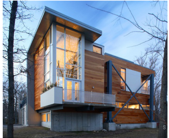
SINGLE speed DESIGN. Big Dig House . 2006. [Online image] Salvaged pieces of the interstate were used to frame the structure for this Cambridge home.
